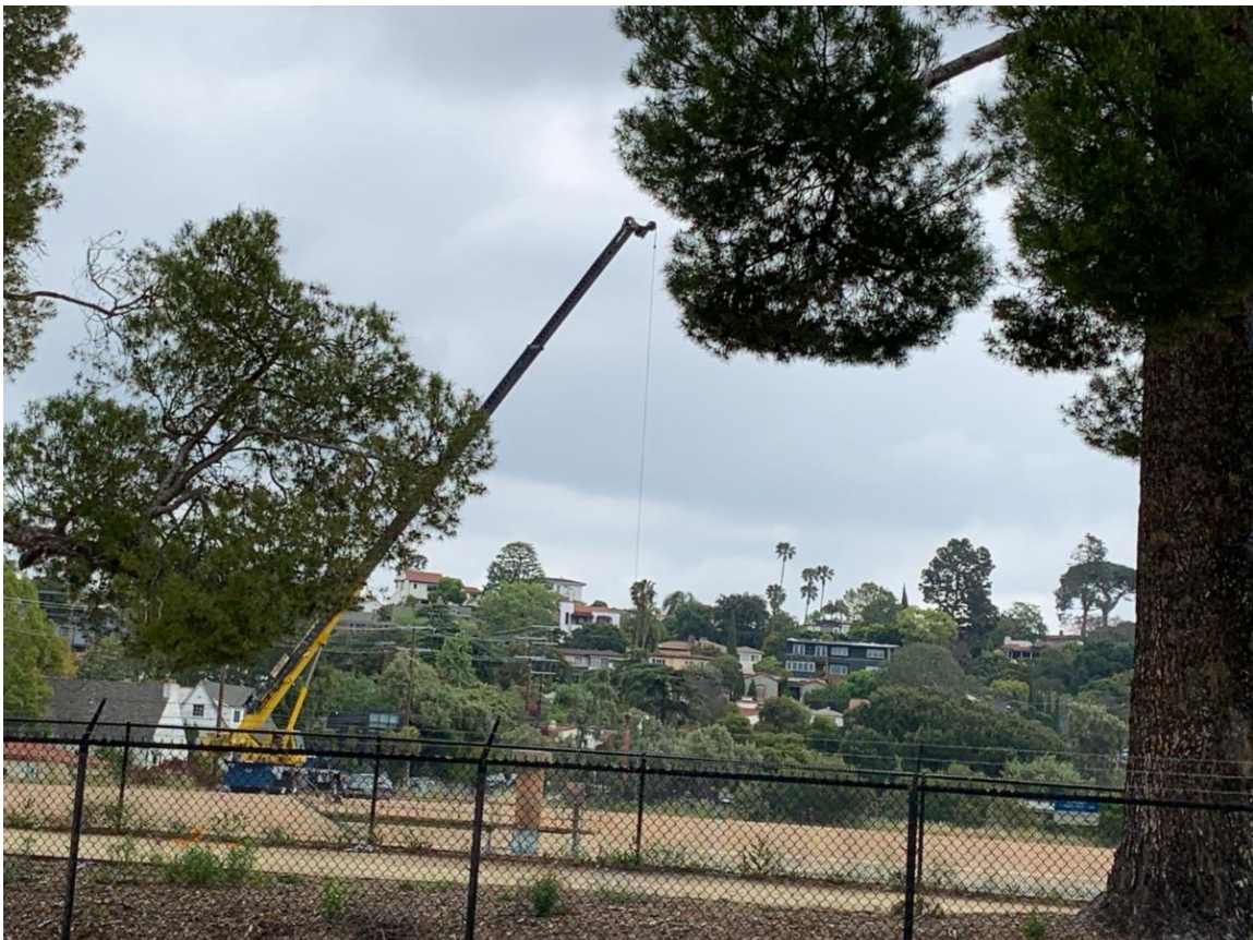
LADWP continues work on the reservoir aeration project.
